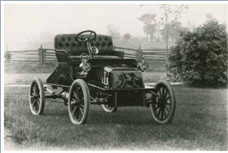
1903 Auburn, single-cylinder engine that produced six horsepower.
