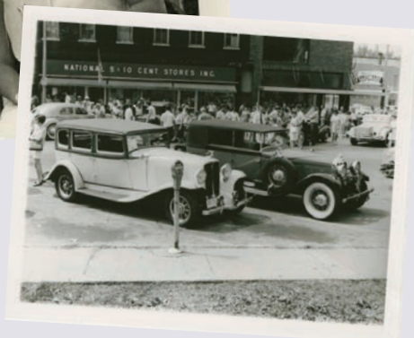
RIGHT: Cars parked at the Courthouse post-parade
